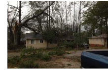
Submitted Tornado Damage
