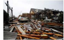
Monday Tornado Damage-1
