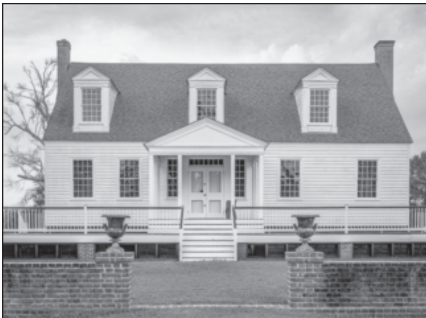
Figure 1. South facade of Batchelor House with archaeologically reconstructed central porch
