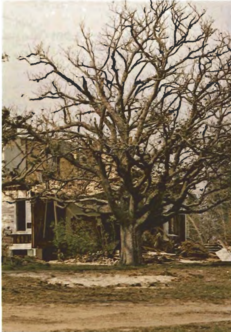
Figure 4. Damaged home and live oak ( Quercus virginiana ) along Highway 90 and open waters of Mississippi Sound at Long Beach, Mississippi.
