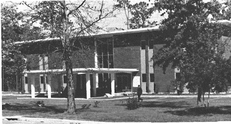
Figure 1. The Richard L. Caylor Building, completed in May 1971, was constructed with $466,000 appropriated in 1966 by the Mississippi Legislature. The facility contains a total of 17,000 gross square feet. Usable space is occupied by The Gunter Library, that houses the Laboratory's extensive collection of literature in the marine sciences, by classroom and research laboratories and by large lecture rooms.
