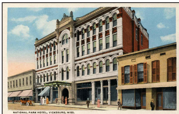
Exterior of the National Park Hotel, Undated. 99
