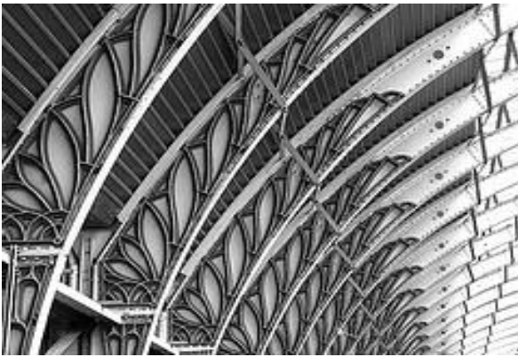
Figure 2: Arched Trusses at Paddington 86
