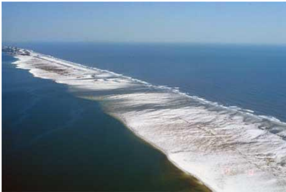
Figure 4: A breach of the Santa Rosa Barrier Island after the impact of Hurricane Ivan (NOAA).
