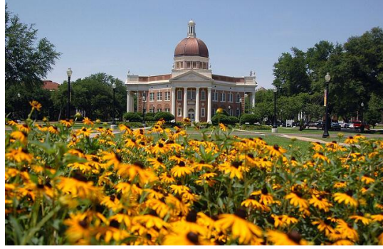
Figure 5.4: Clean, complete Administration Building image.
