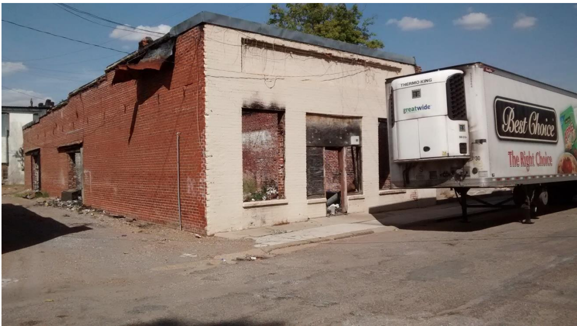
Illustration 3. Prior to a shift in political power to African Americans, Shaw was prosperous community with a thriving downtown business district. Following white flight, the majority of the downtown buildings are abandoned, like this one, and in various stages of deterioration.
