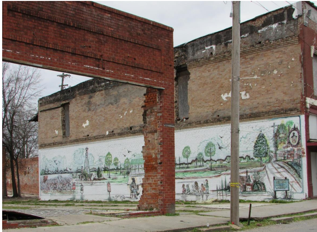
Illustration 5. The once upscale store adjacent to DHH is now simply the remnants of its storefront and a portion of the interior floor of ornate gray and white ceramic tiles.
