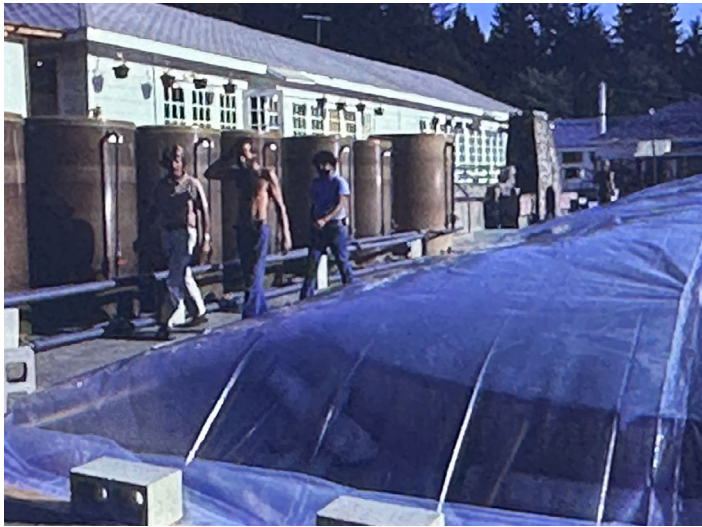
FIGURE 5. The Aquaculture Research Center in the redwoods of Boulder Creek, CA where we conducted Spirulina culture research. The facility was previously used as the town swimming pool. The pool for algal culture is underneath the plastic sheet in the foreground. The fiberglass tanks stored the chemicals and nutrients to grow the algae. The snack bar which was renovated into the laboratory is in the background behind the fiberglass tanks. The individuals in the photograph worked at the algae culture facility.
