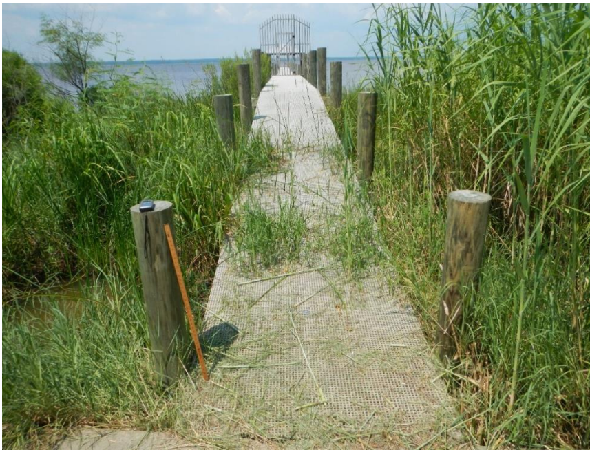
Figure 19: Image of pier at site HAN-06-A.
