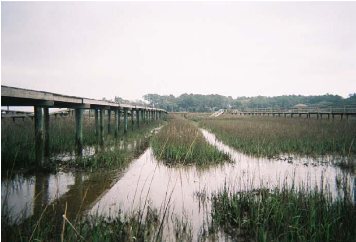
Figure 14: Image of heavy equipment damage at site HAR-05-B in 2006.
