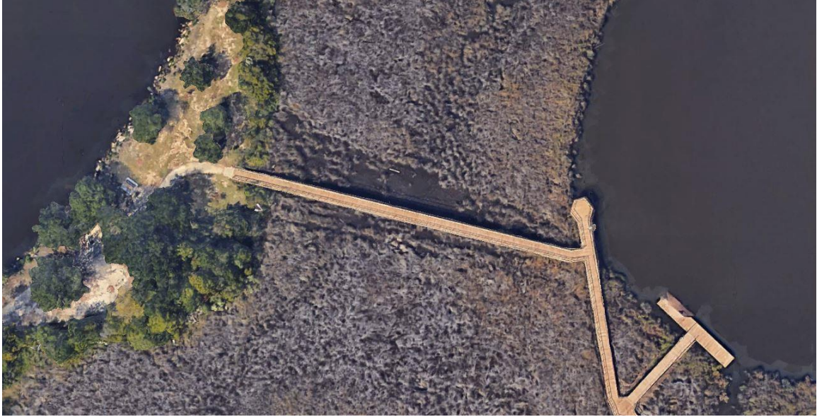
Figure 17: Aerial image of heavy equipment damage at site HAR-05 (Google Earth).
