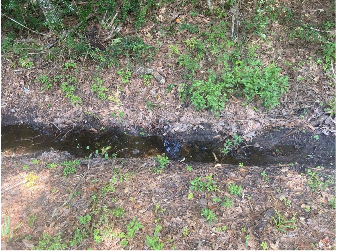
Figure 2.2 Rainwater ditch found in St. Tammany Parish, LA
