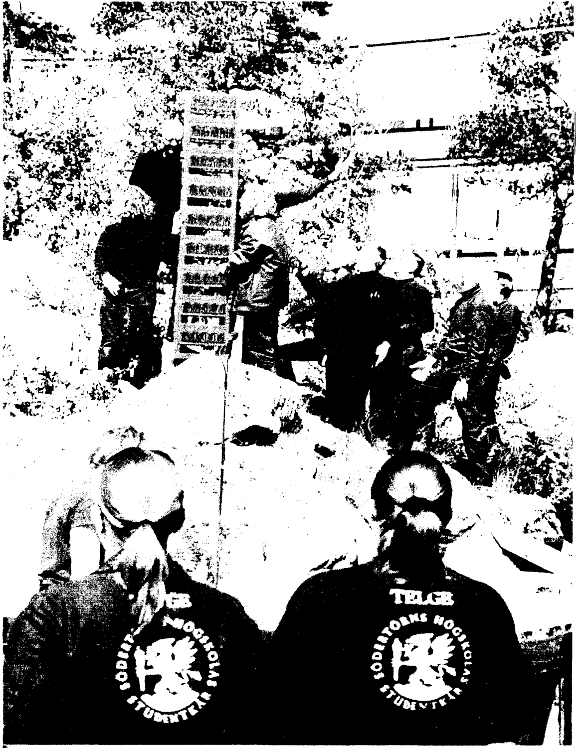
Figure 4. Reenactment of a Stage in the Construction Process. The crates symbolize Moas Båge. The rocks and some trees have been preserved in the middle of the campus.
