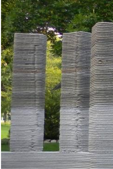
Figure 5.14 Extrusion End Points in Aligned Pattern
