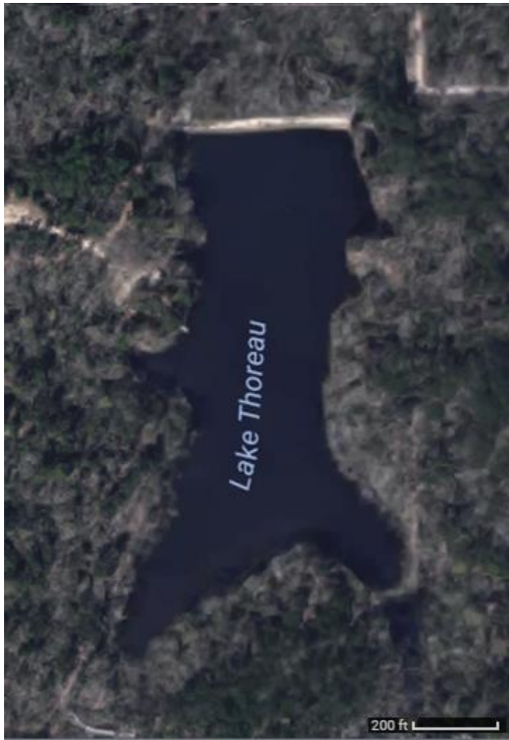
Figure 1. Lake Thoreau aerial view (Google Maps).
